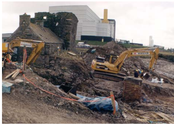
Figure 3 Beginning the remediation of Downreay Castle
