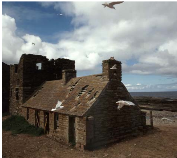
Figure 4 Downreay Castle after remediation
